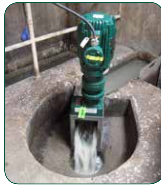
Muffin Monster with immersible motor
