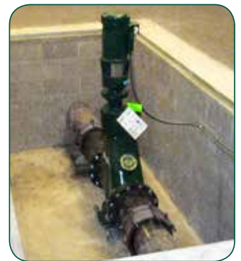
Muffin Monster in-line grinder in a prison
