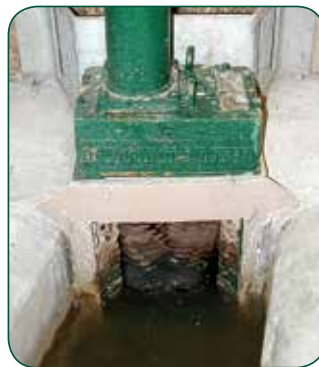
Muffin Monster channel grinder in a prison
