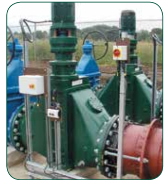
Macho Monster in-line sludge grinders
