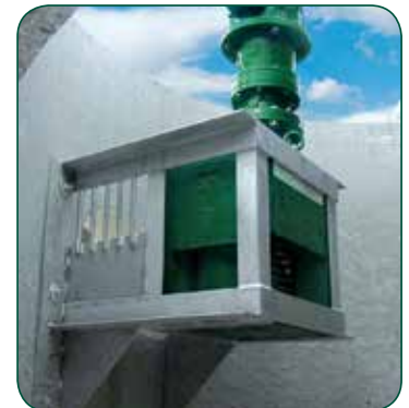
Mini Monster installed in a pump station
