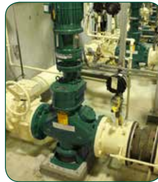
Muffin Monster in-line sludge grinders
