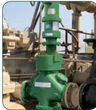
Muffin Monster in-line sludge grinder
