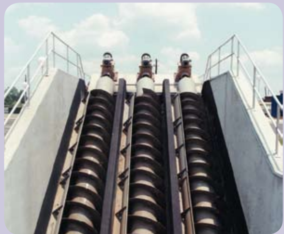
Open Flight Screw Pumps with sizes from 20” to 108” in diameter. Lift capability up to 30’.
